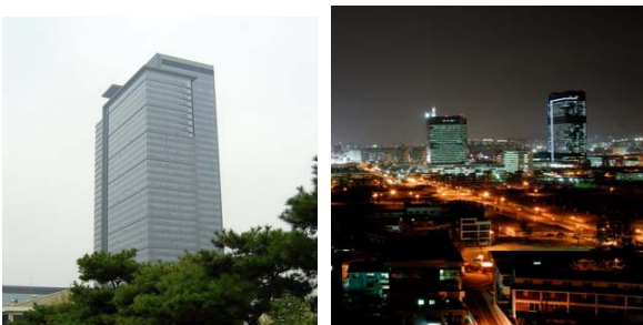
Fig. 1 View of building A and B
