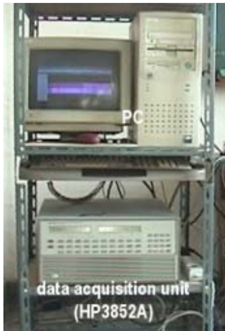
Fig. 12 Data acquisition unit
